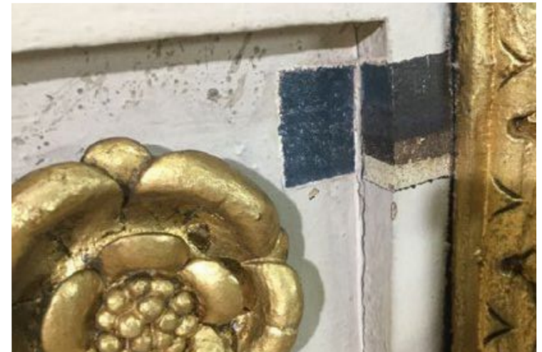
FIG. 19 Detail of an uncovering trial in the coffer soffit, north-east corner of Union of Crowns , showing 19th-century blue background.
