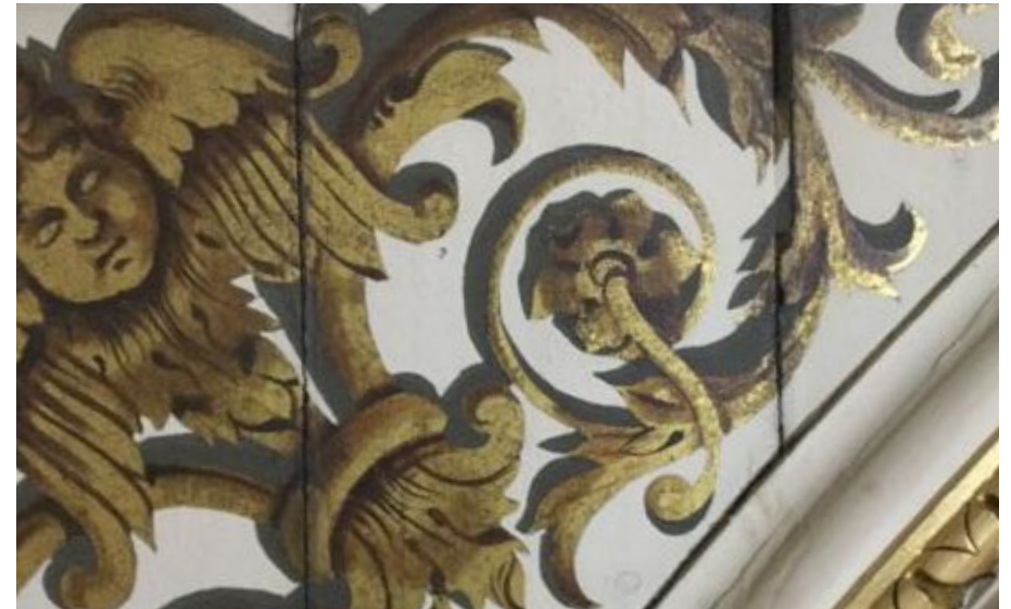
FIG. 7 Detail of the south-east spandrel caisson of Apotheosis , showing the visible planks of the original timber support.
