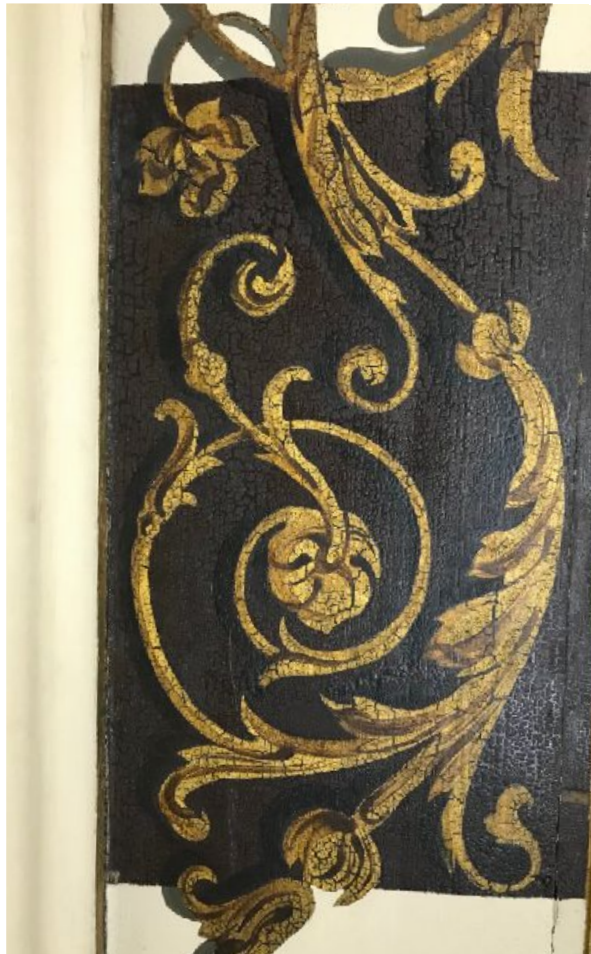
FIG. 6 ABOVE Detail of an uncovering trial on the planceer at the north end of the ceiling, revealing Soane's scheme. Note the dark shadows, which offer much more contrast with the gilding than the modern, opaque, greyish shadows visible at the top of the image.
